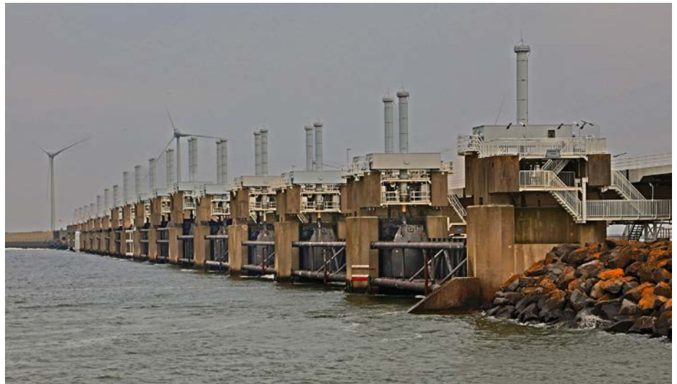
The Delta Works in The Netherlands, a well-known example of a public good, has been declared one of the Seven Wonders of the World by the American Society of Civil Engineers.
